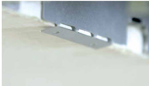
Securing tabs press against the sheetrock, securing fan in place
